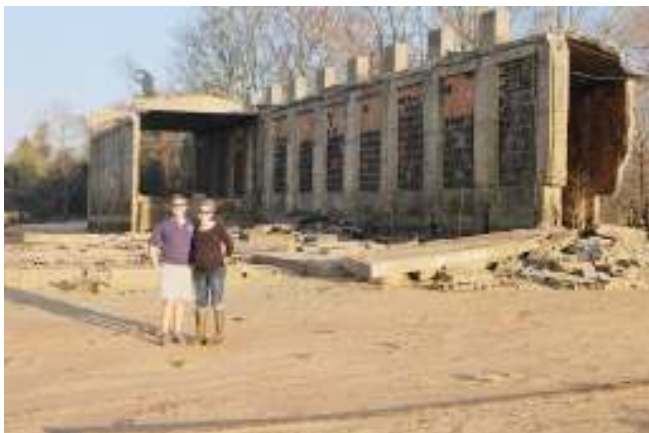
Seth and Patty in front of the remnants of dry kiln
