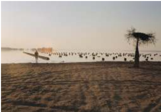
Foundation of the sawmill
